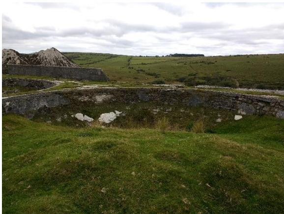
Alongside the pits were the mica drags (popularly known as 'micy drags' in local Cornish dialect). These stone lined channels, set in the ground, were where the clay in slurry form was pumped from the pit. The heavier micaceous waste material would settle out, after which men would scrape (drag) along the lines to remove the waste material before the clay was channelled into the settling tanks. The building in the background would have been the Pit Captain's House.
